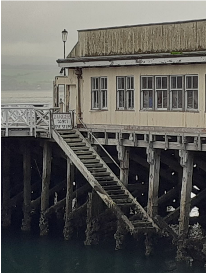
Image B2.1 Victorian Pier, south side, steps not in use
